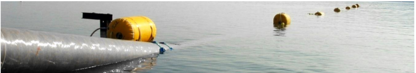
Water pipe going 5 km on the bottom of Geneva lake
