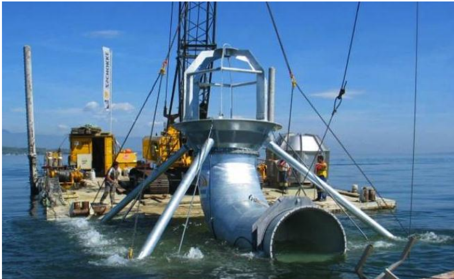
Water pipe going 5 km on the bottom of Geneva lake
